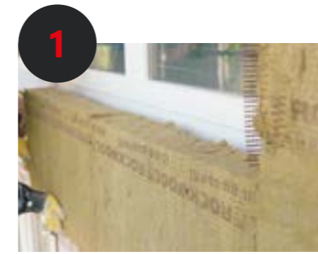
1 Application of insulation panels to the facade
