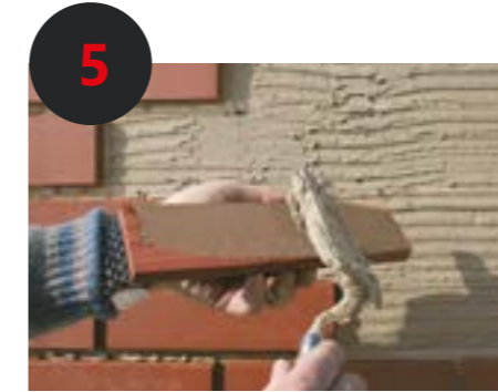
5 Application of adhesive to the slip (buttering-floating procedure)
