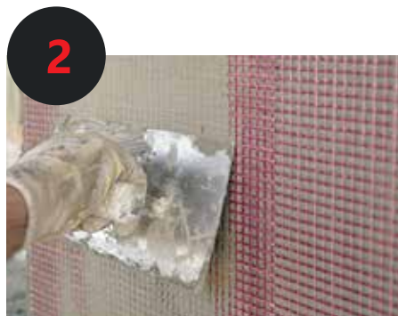
Installation of a reinforcement layer
