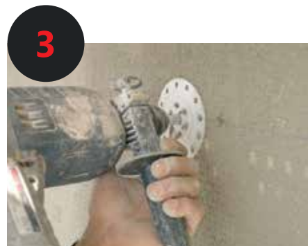
Fastening of insulation panels with special anchors
