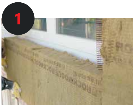
Application of insulation panels to the facade
