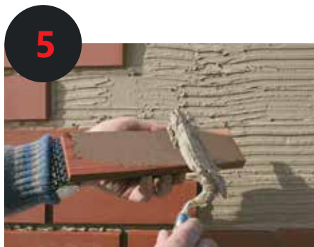
Application of adhesive to the slip (buttering-floating procedure)
