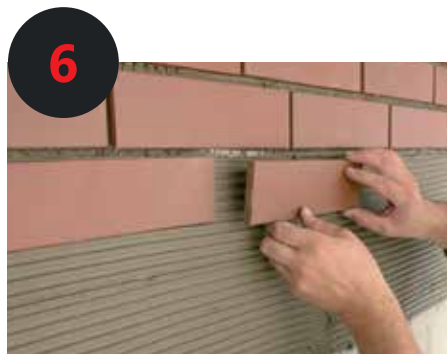
Setting the slip in the adhesive
